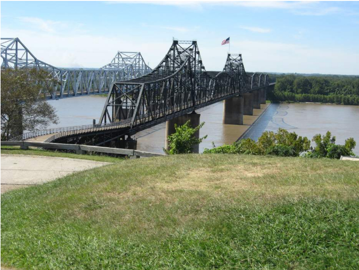
U.S. 80 Mississippi River Bridge with I-20 Bridge in Background
