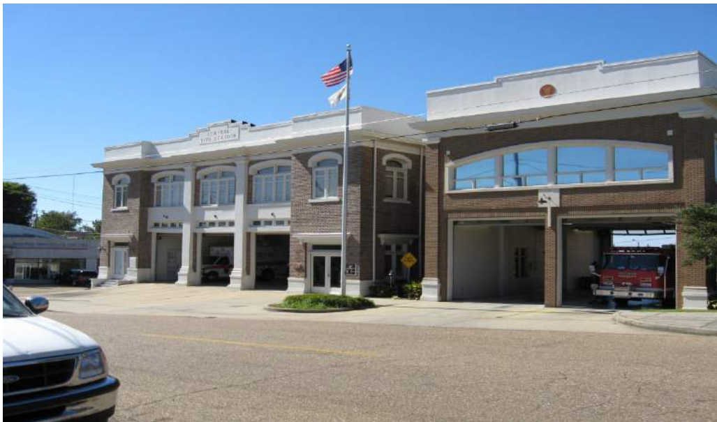
Central Fire Station
