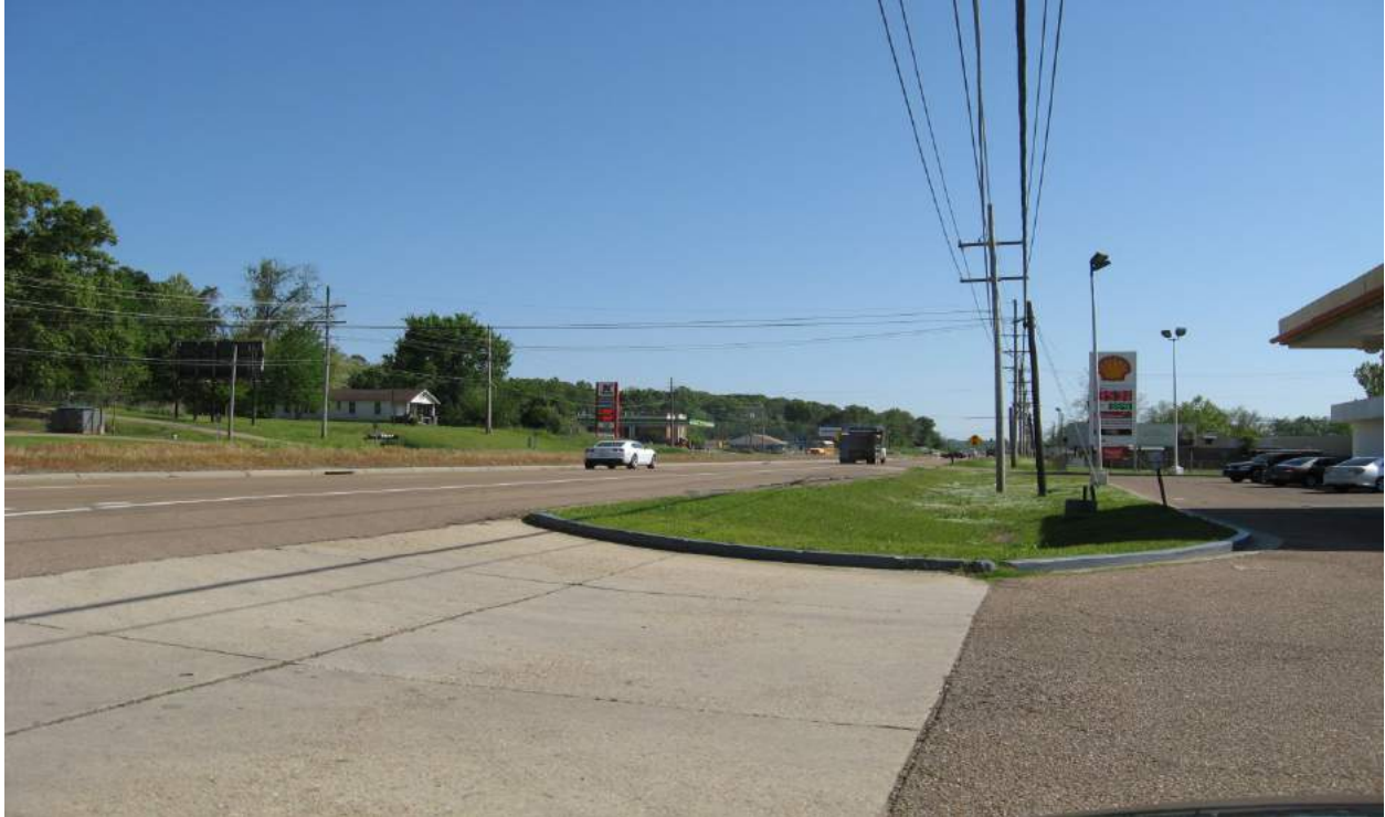
View of U.S. Highway 61 South
