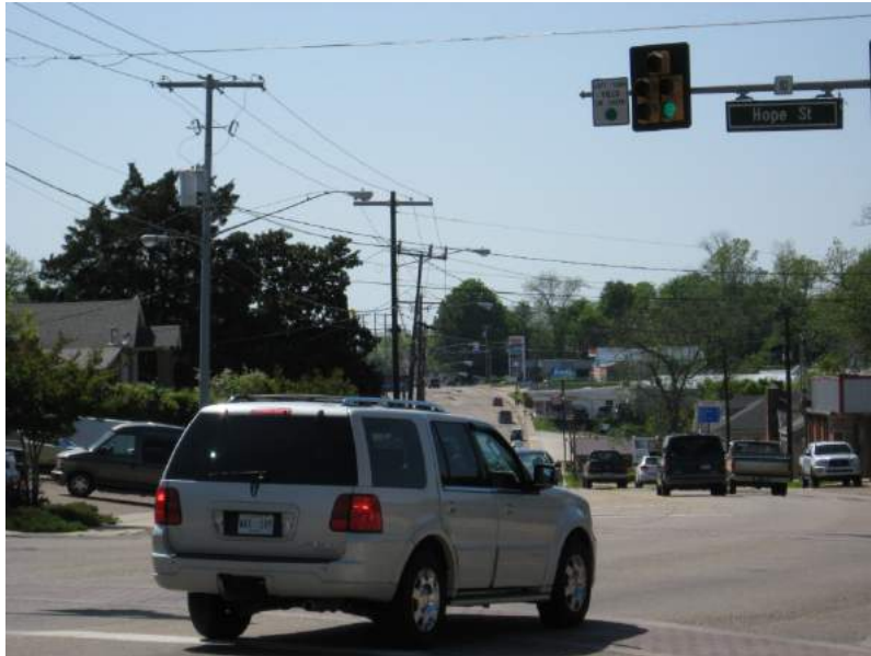
Current View of Overhead Wires on Clay Street
