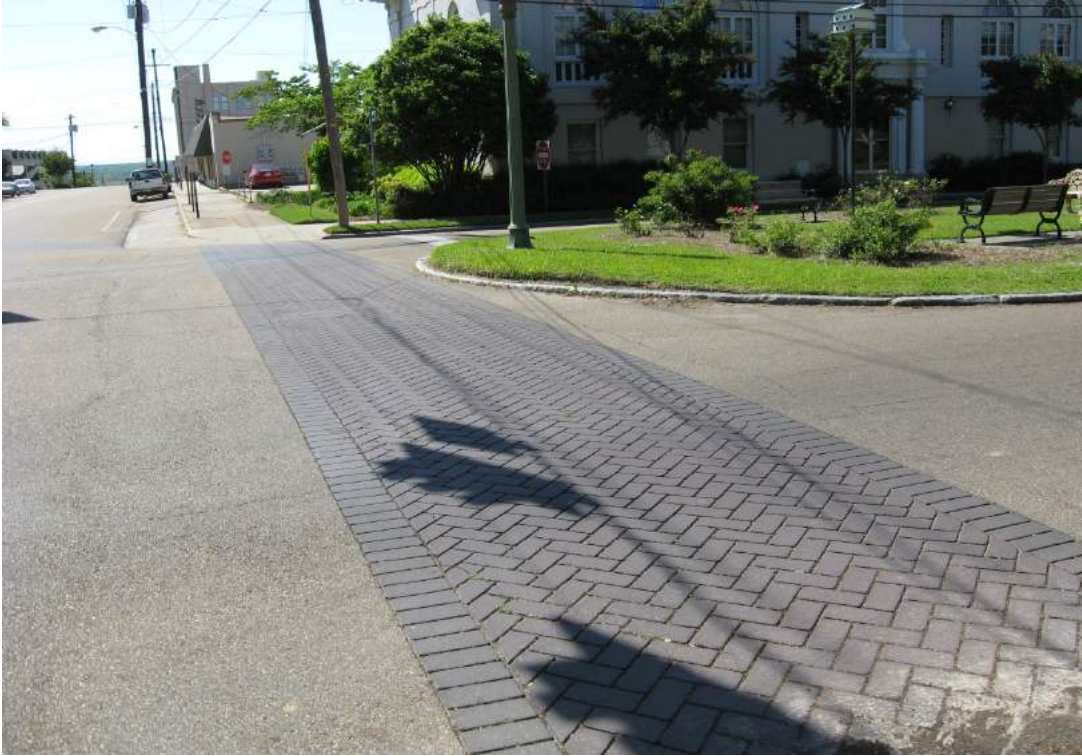
Brick Crosswalks in Downtown Area
