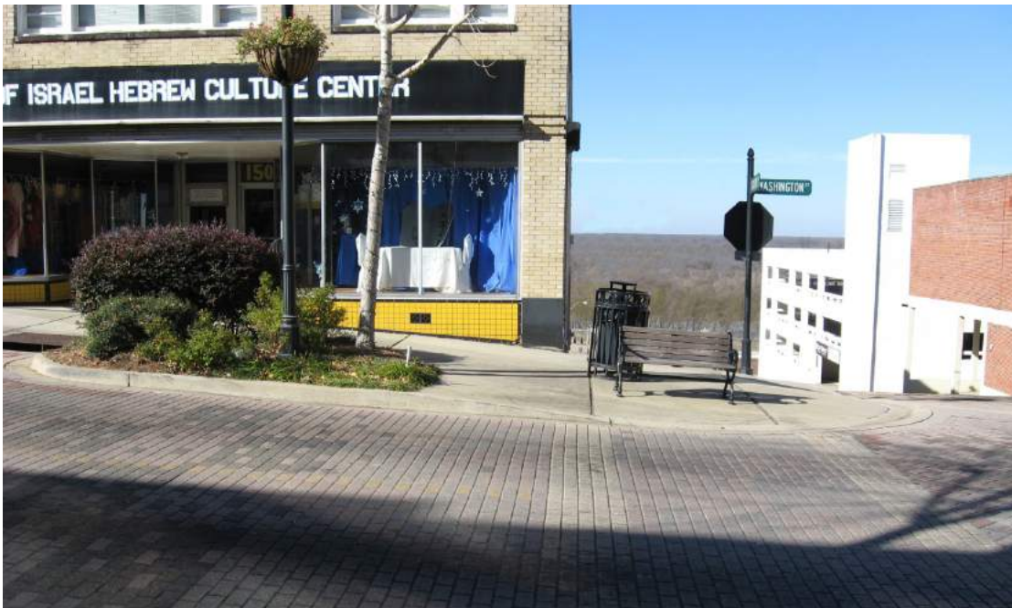
Viewshed at Washington and South Streets without Overhead Power Lines
