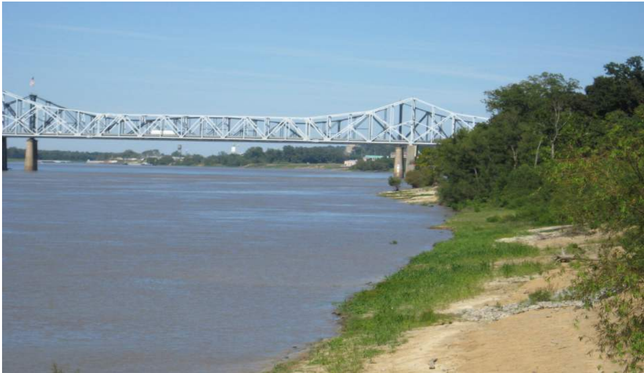
View of Mississippi River Edge with Bridges and Vicksburg in the Background
