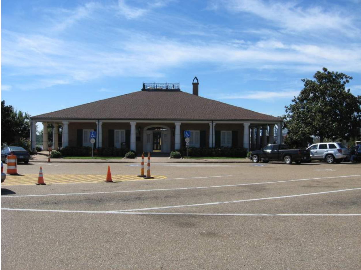
Mississippi River Bridge Visitor's Center
