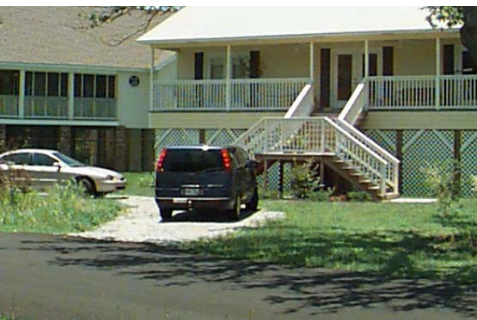
This home is elevated three feet above the BFE.
